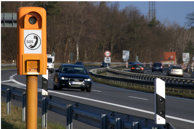
The roughly 16,000 emergency call boxes on German highways are erected in 2,000 meter intervals on both sides of exit and entrance ramps.
