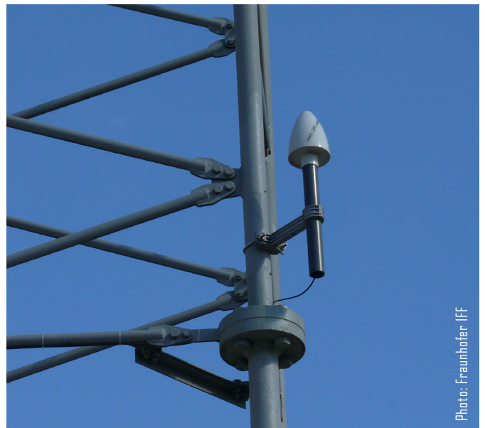
The phasor measurement unit transmits data packets to headquarters by satellite.
