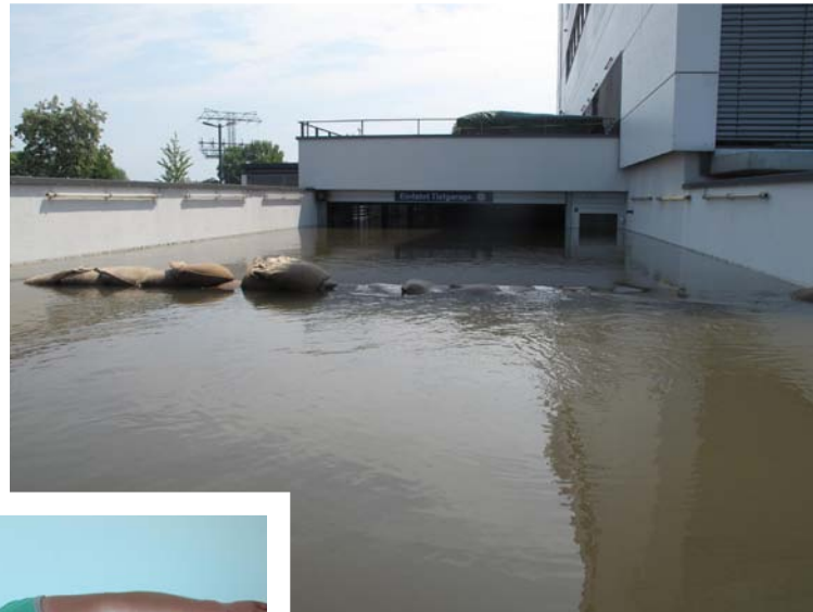
The entrance to the VOTC's underground garage. The water in it reached around 1.90 meters on Sunday.
